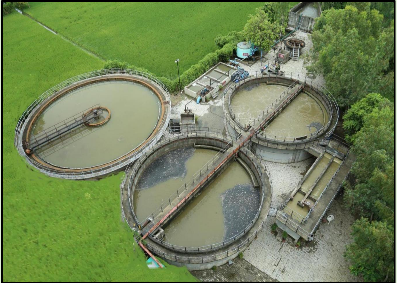
5 MLD Sewage Treatment Plant installed in the campus
