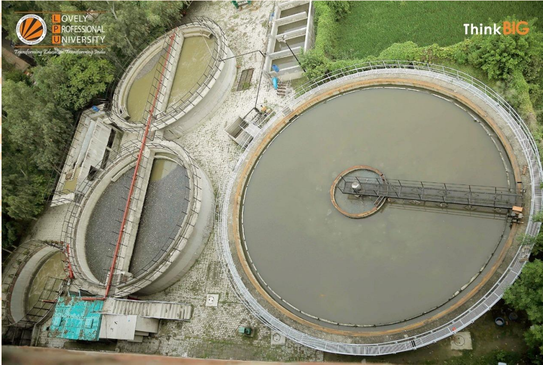
5 MLD Sewage Treatment Plant at LPU
