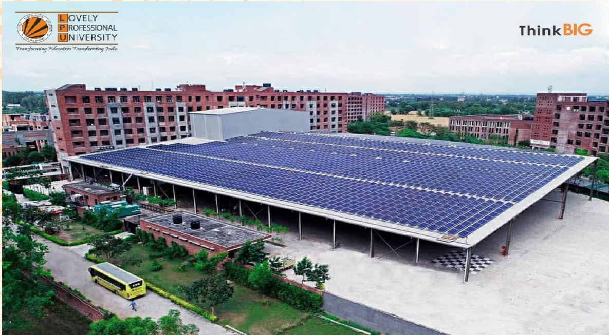
A view of Rooftop Solar PV Plant
